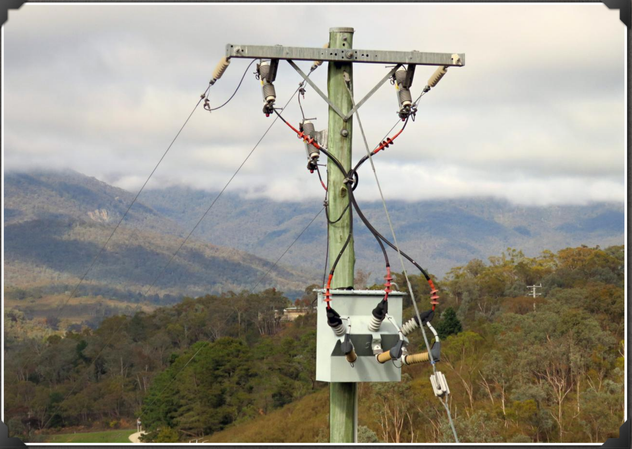
STEP-DOWN TRANSFORMER PRODUCING A LOWER VOLTAGE
