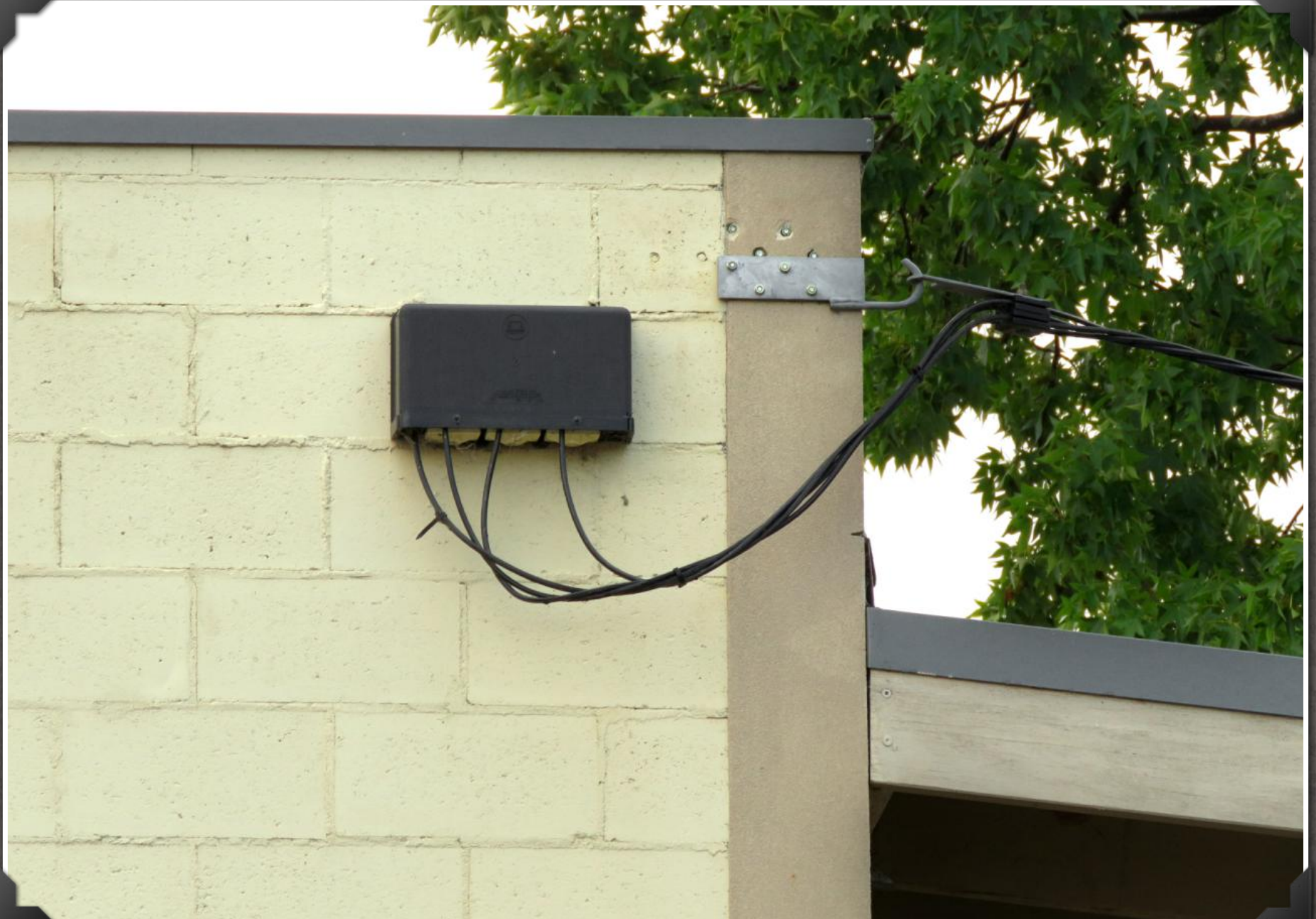
BUSINESS CONNECTION POINT - THREE PHASE POWER (PROVIDING UP TO 415 VOLT)
