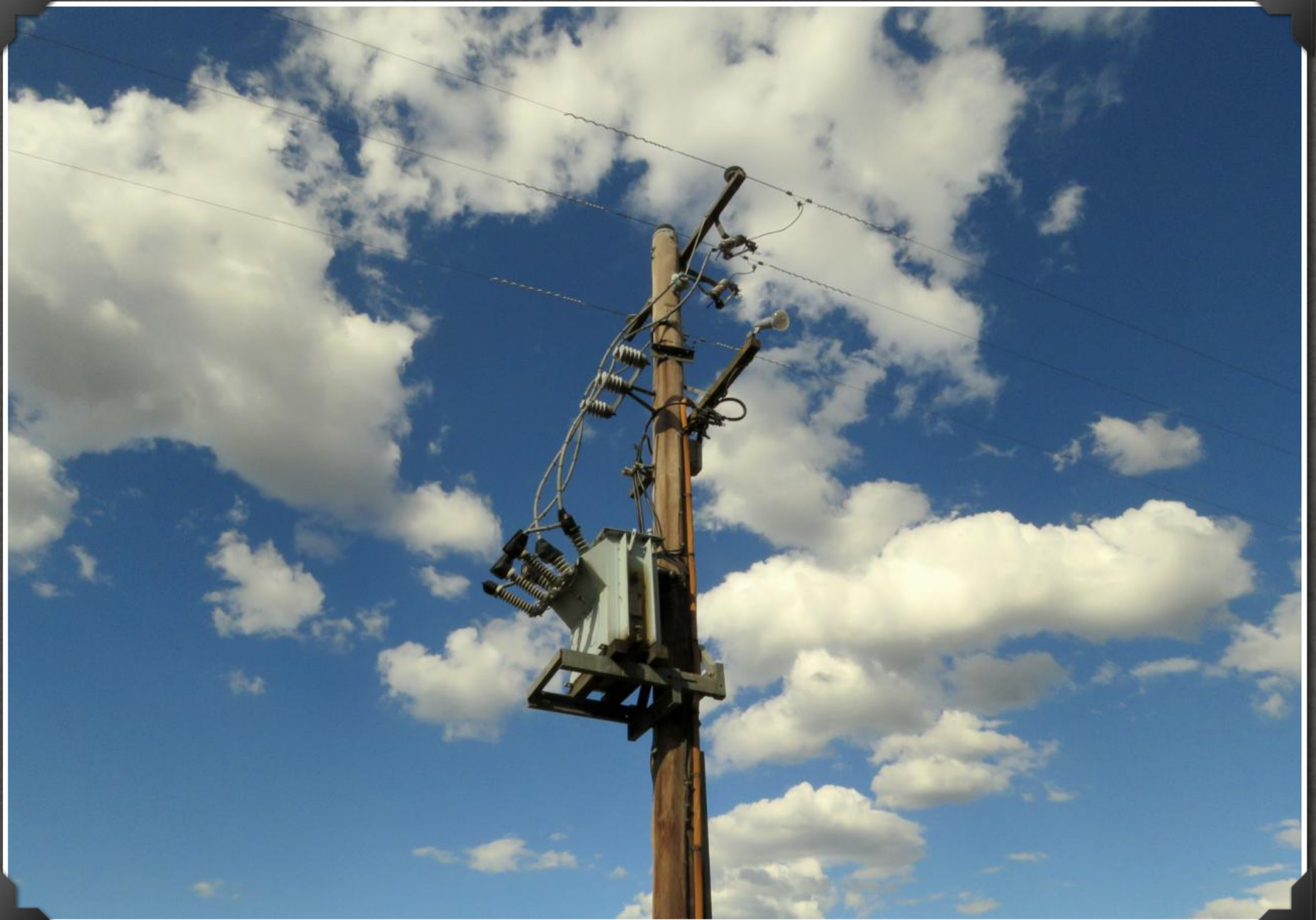
STEP-DOWN TRANSFORMER PRODUCING A LOWER VOLTAGE
