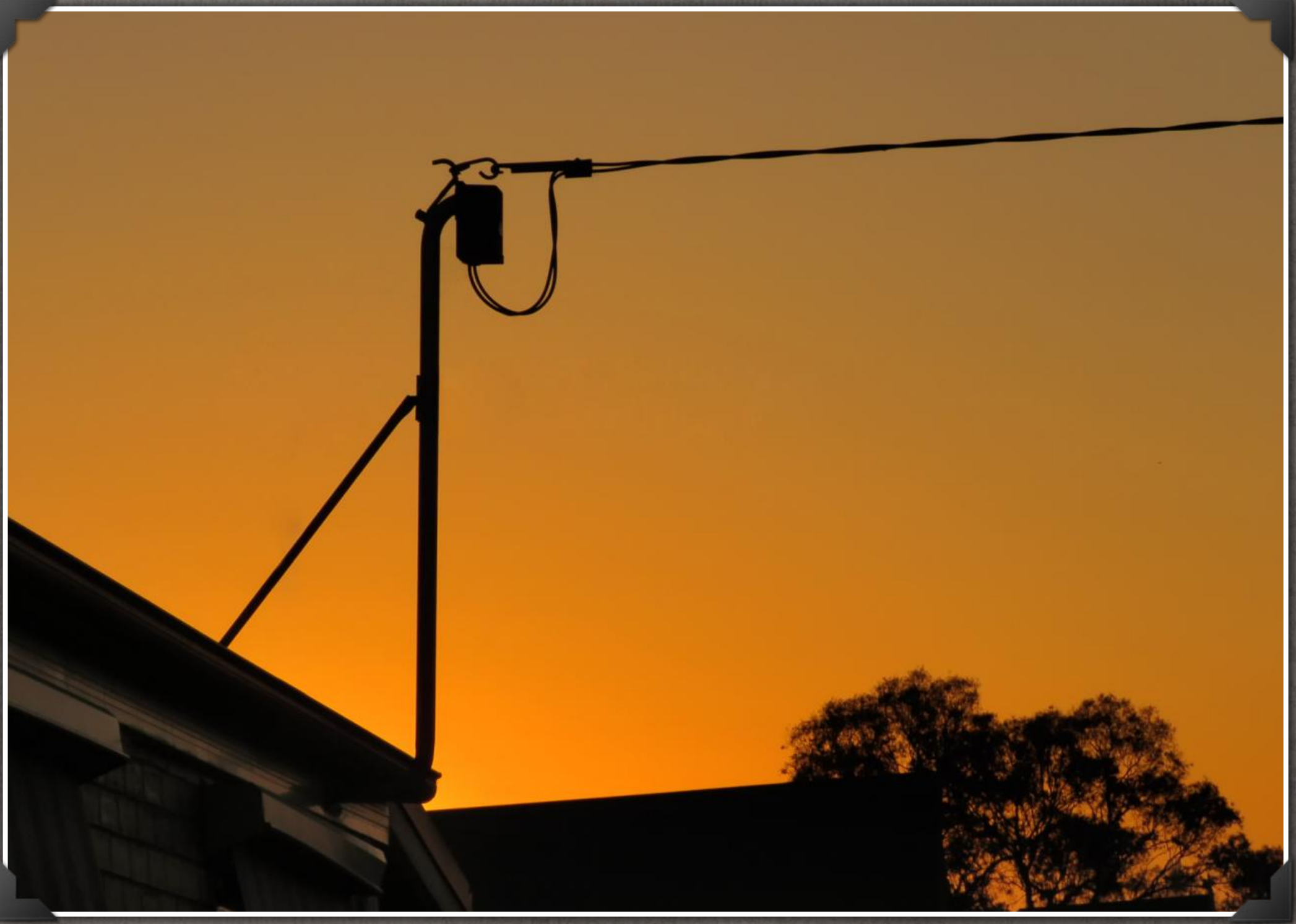
HOUSEHOLD CONNECTION POINT - SINGLE PHASE POWER (240 VOLT)
