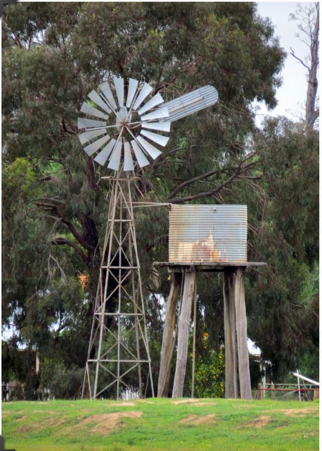
Water is pumped from a local water source to the elevated water tank.
