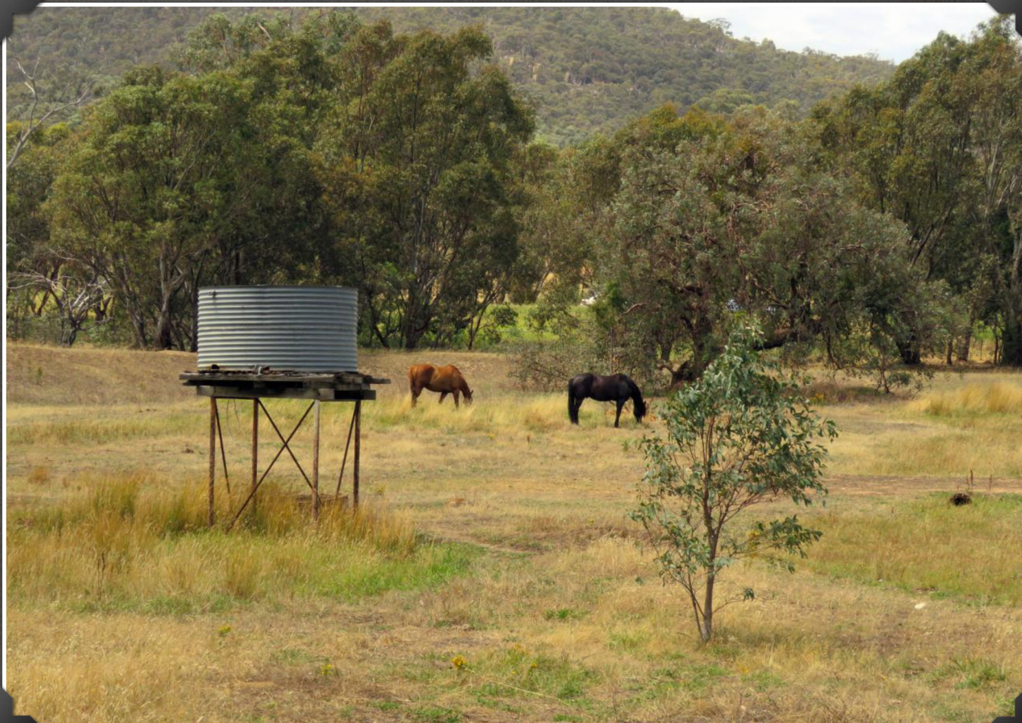
GLENROWAN WATER TANK IN 2017
