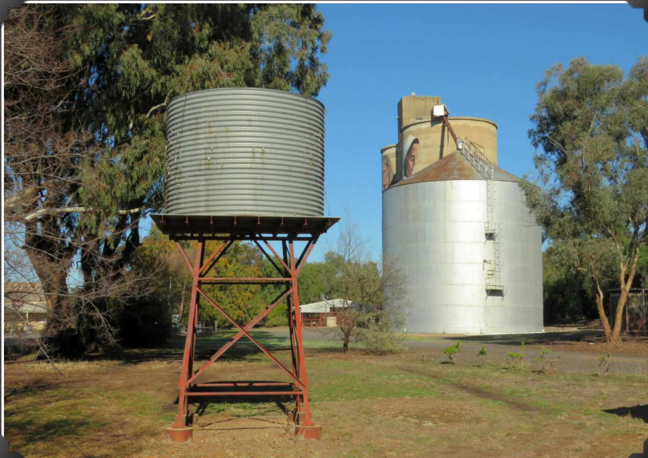
DEVENISH WATER TANK IN 2017
