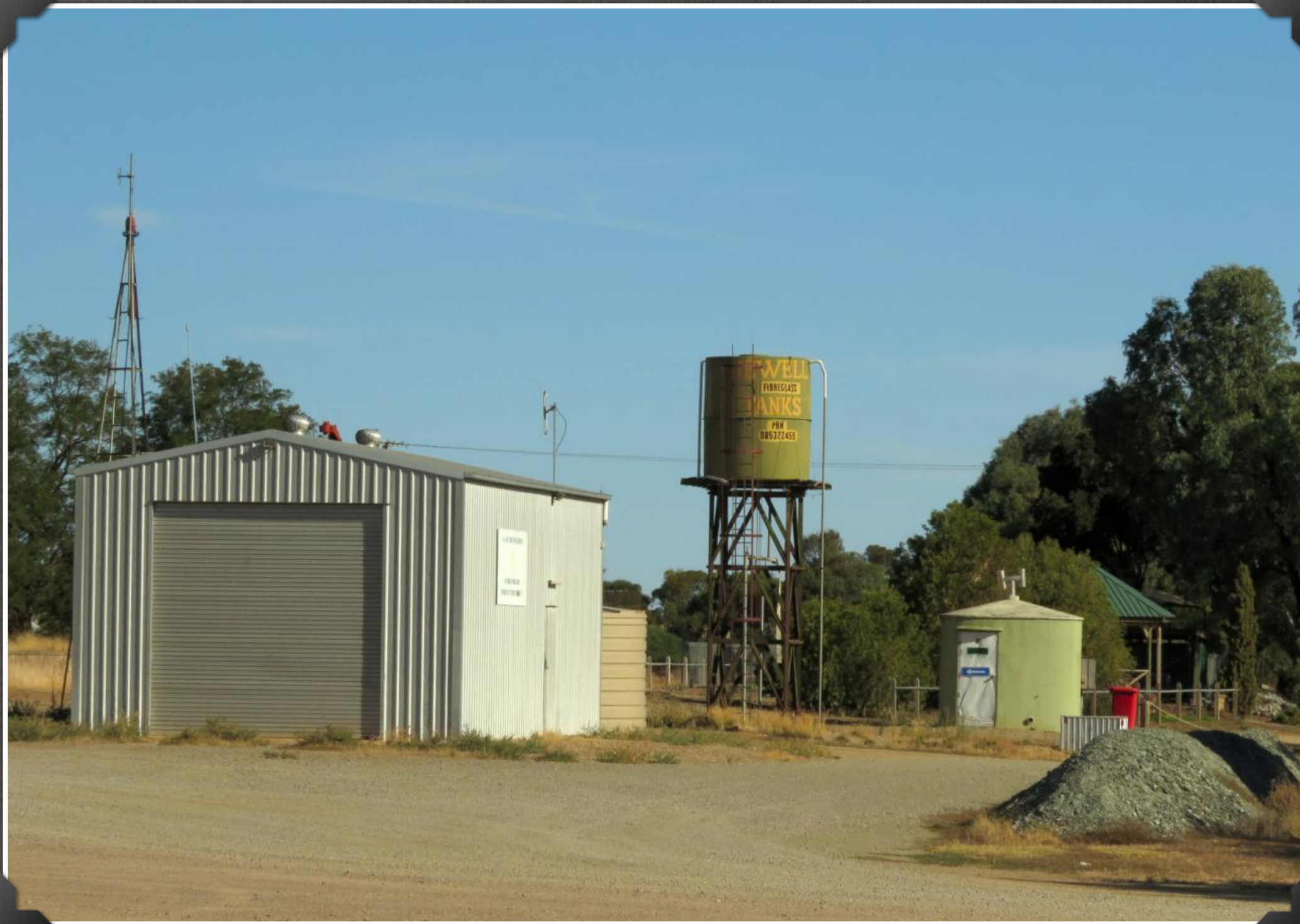
MOUNT BRYAN, SA, WATER TANK IN 2019
