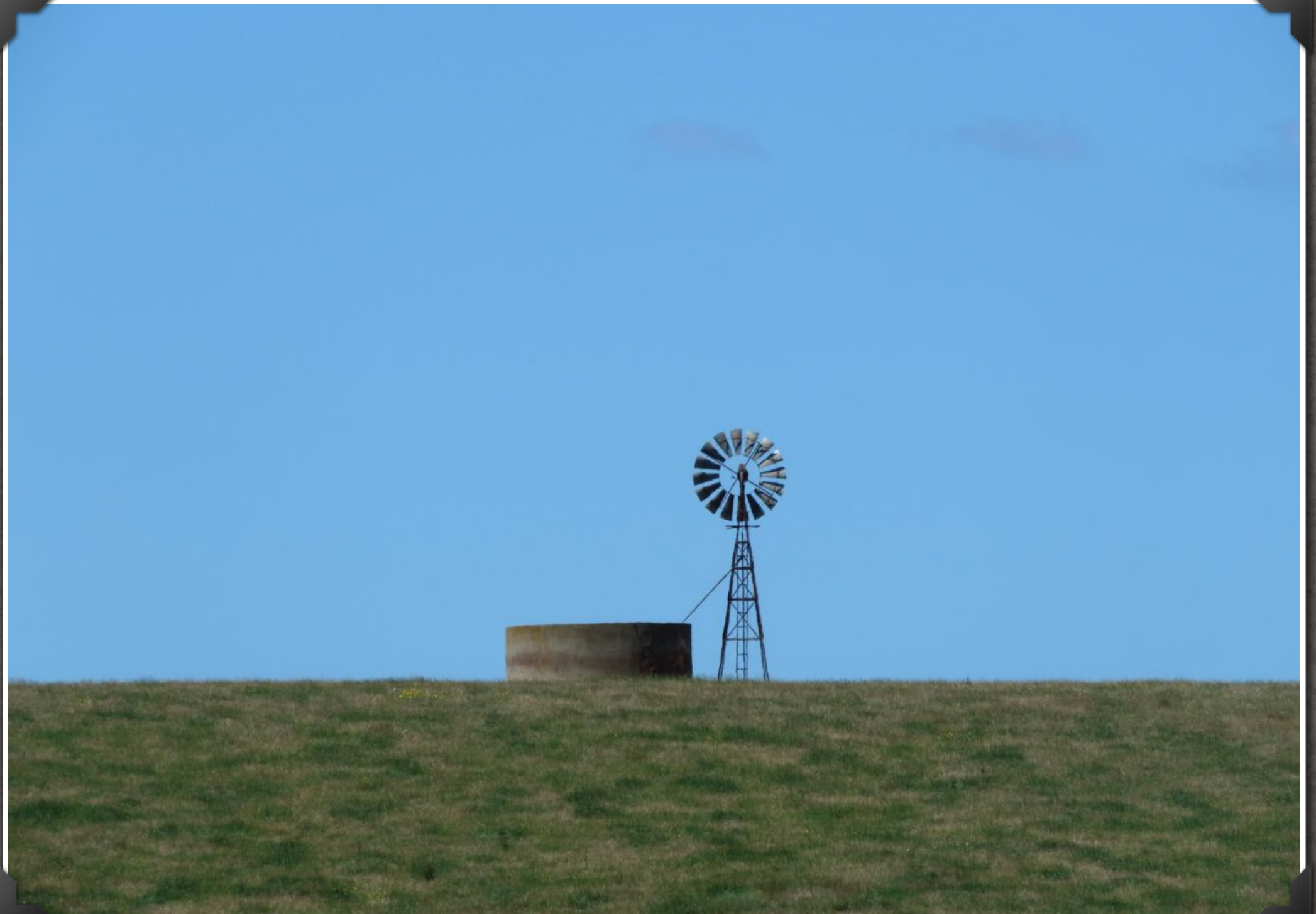
TOOLANGI WATER TANK IN 2018
