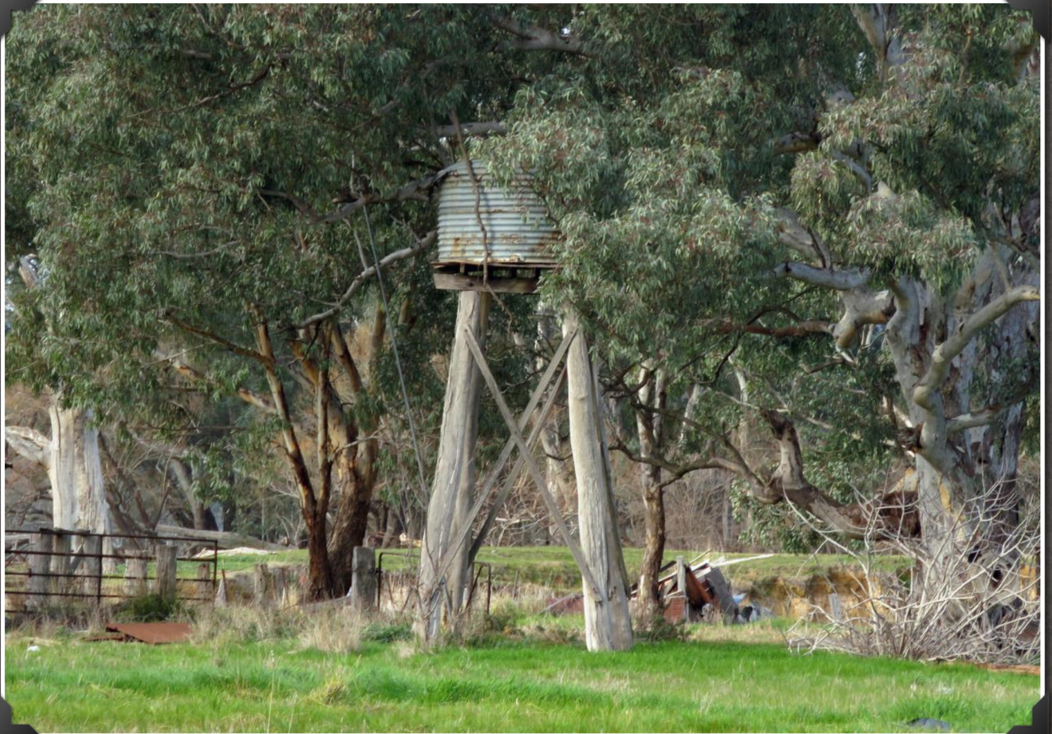
WHITFIELD WATER TANK IN 2018
