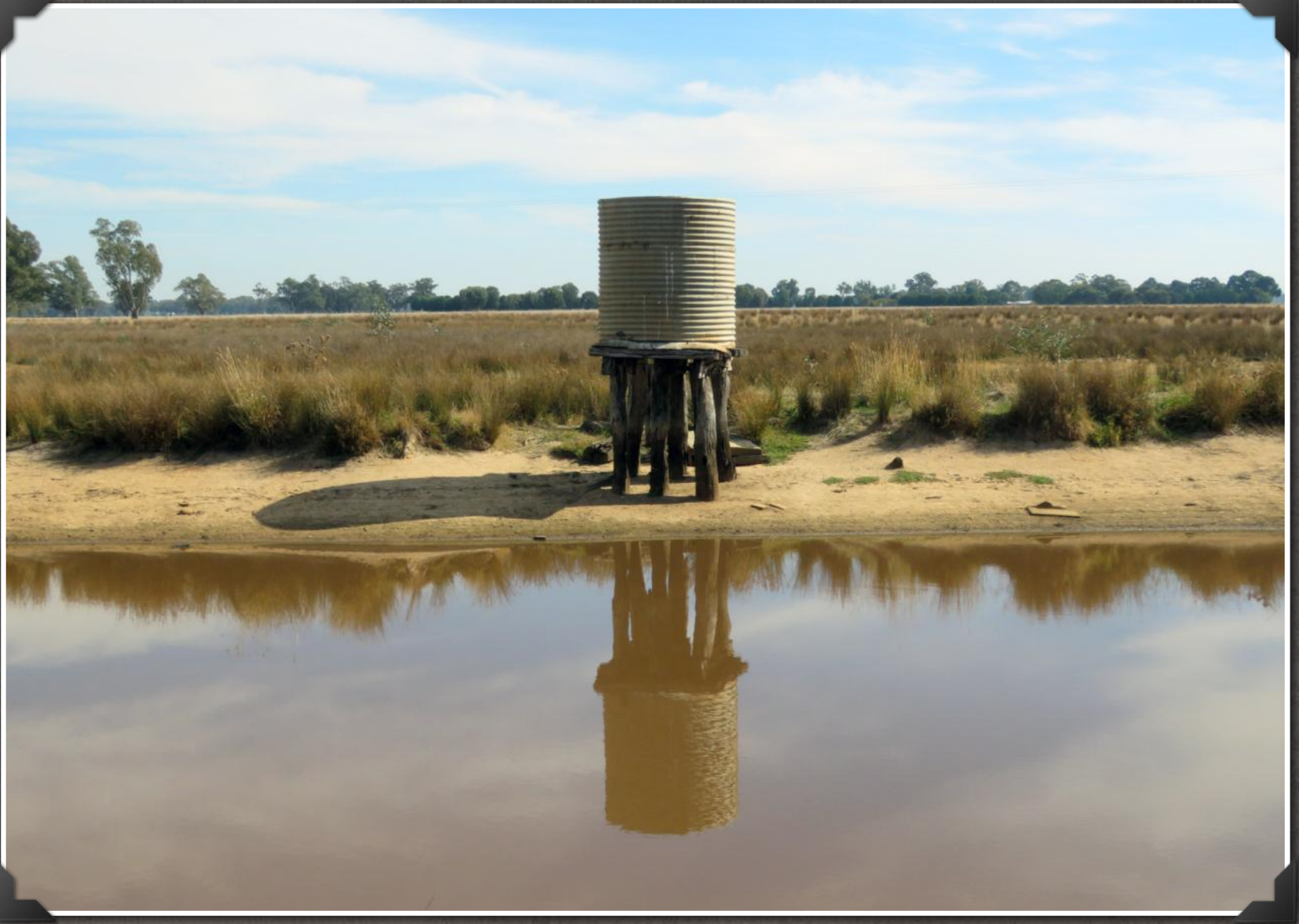
AVENEL WATER TANK IN 2017
