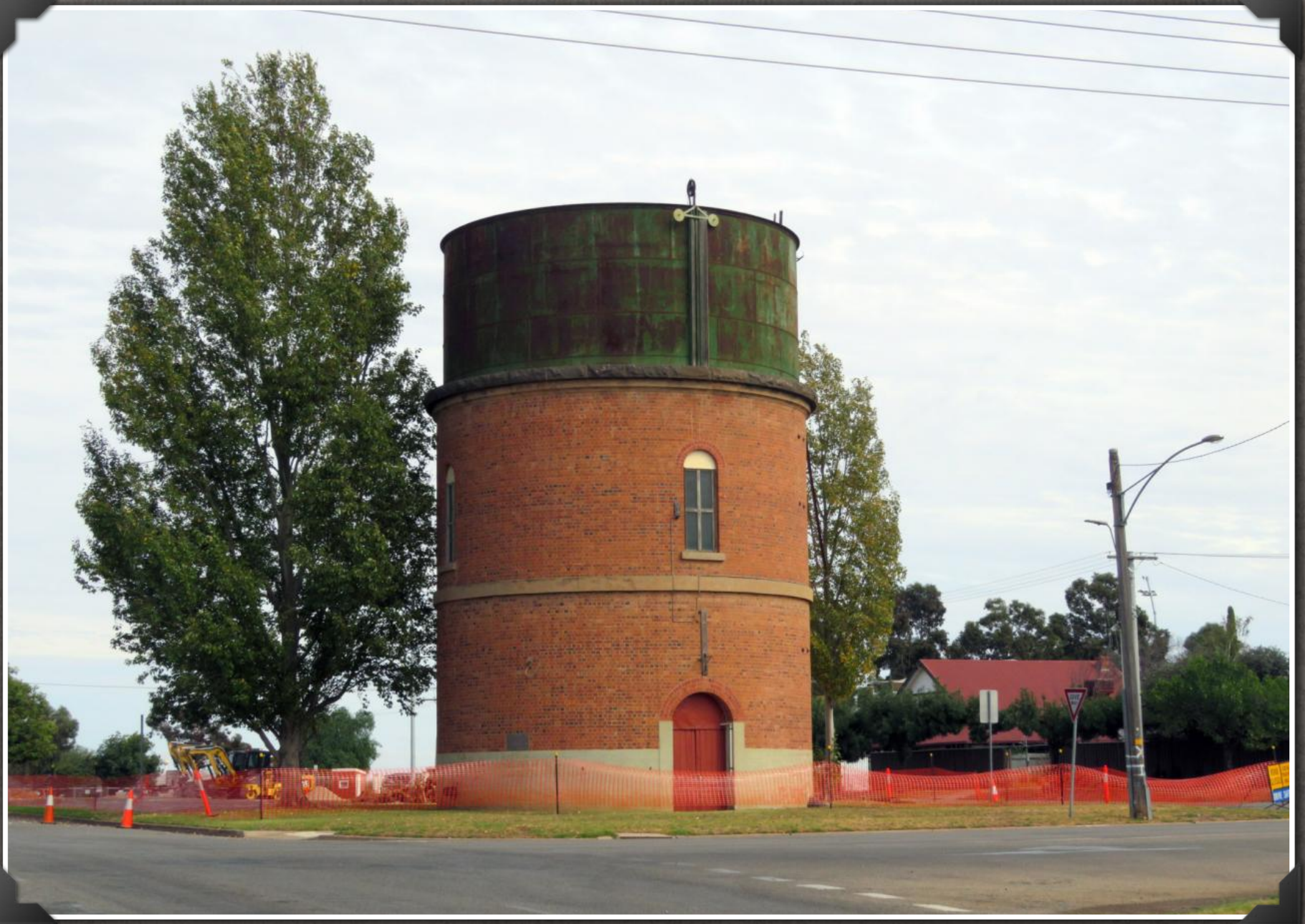
ECHUCA WATER TANK IN 2019
