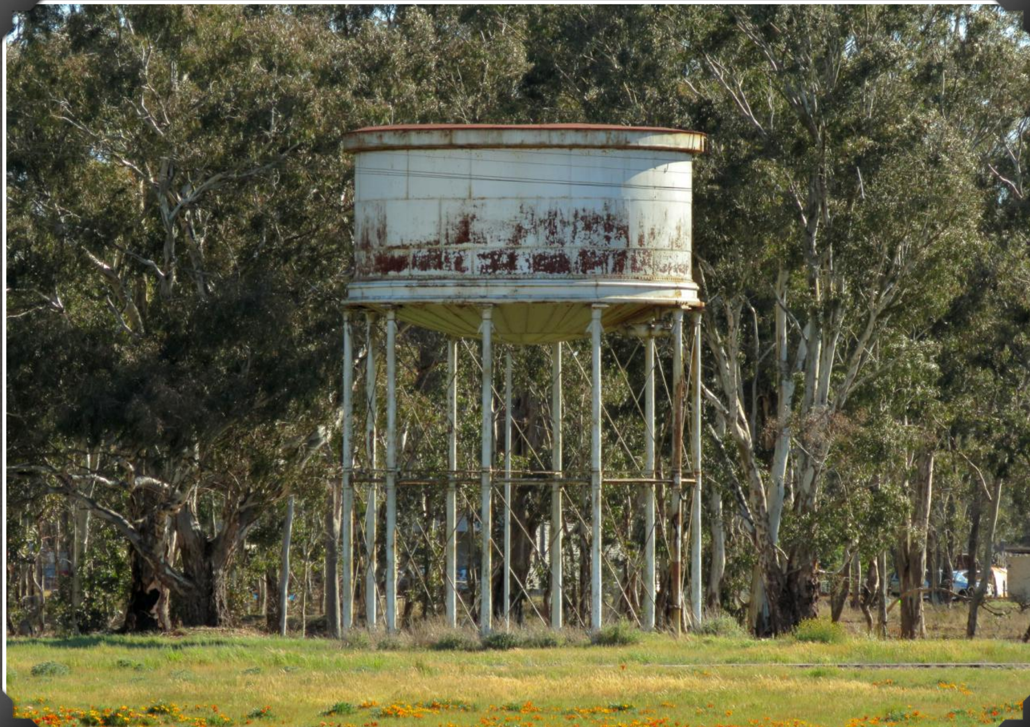
BEALIBA RAILWAY STATION TANK IN 2018
