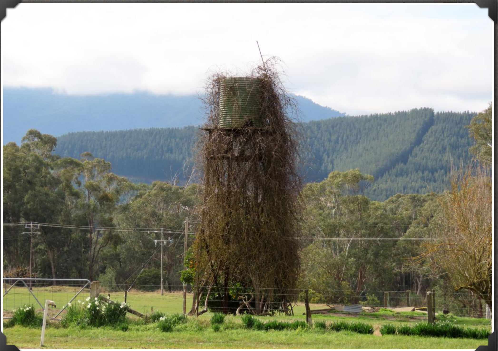
BRIGHT WATER TANK IN 2019
