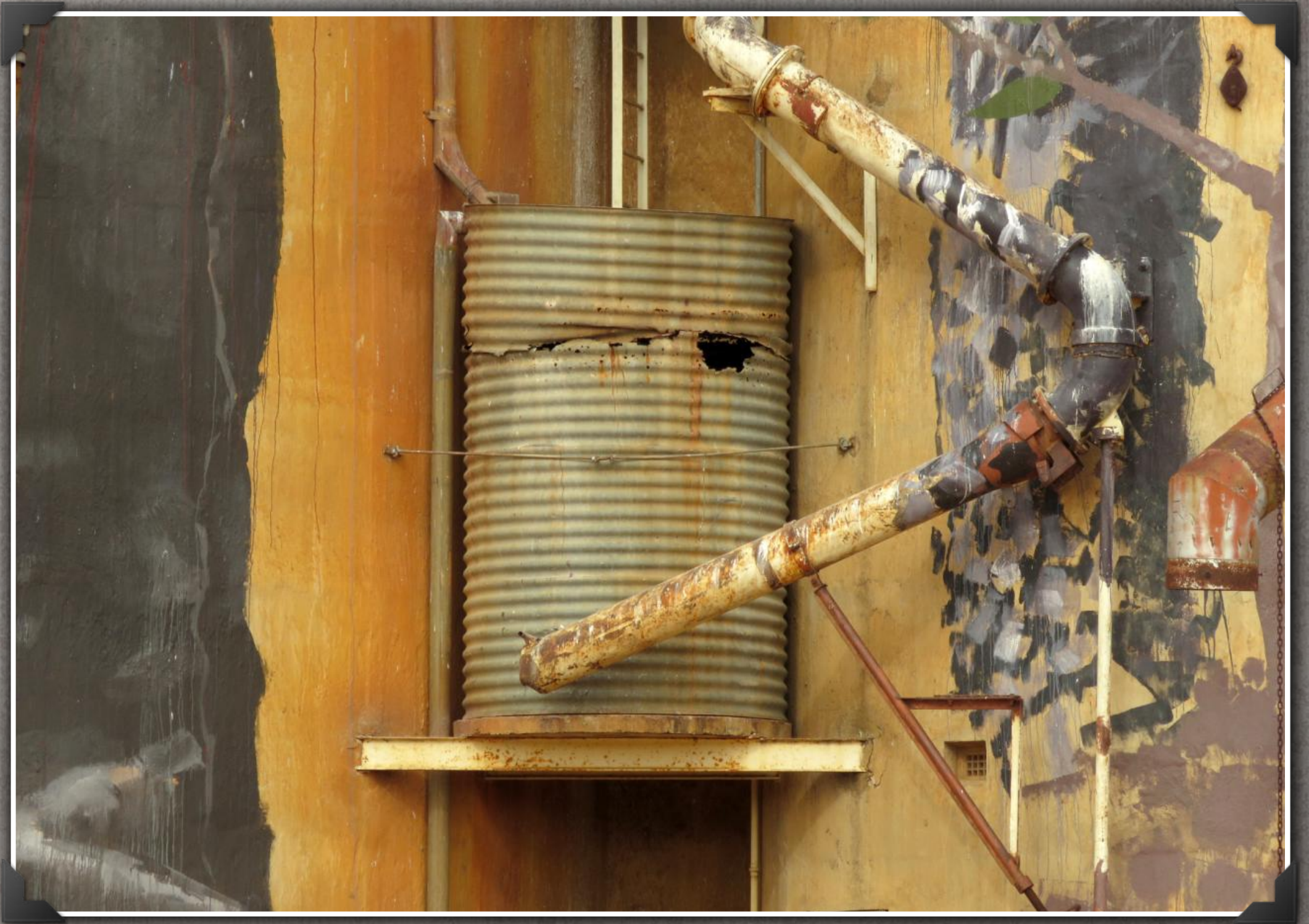
SILO WATER TANK IN 2018
