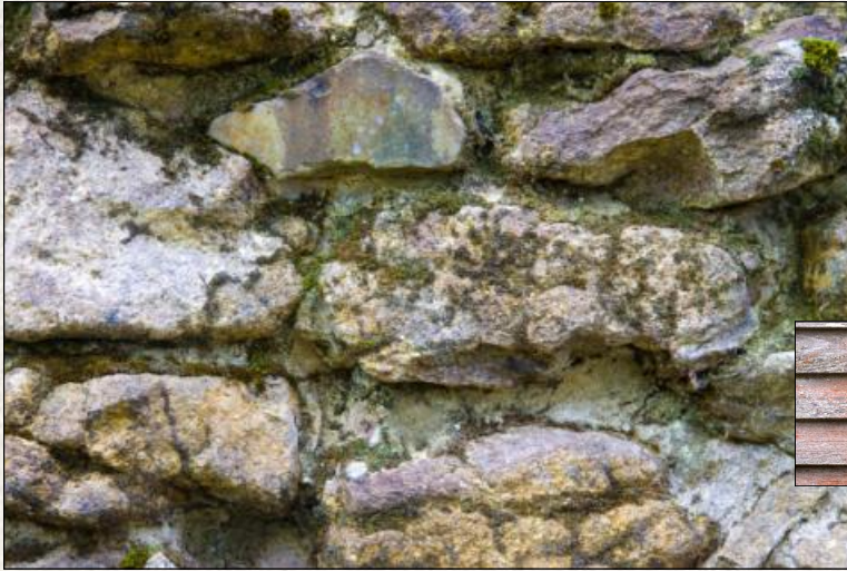
The fireplace was made from local granite in 2008
