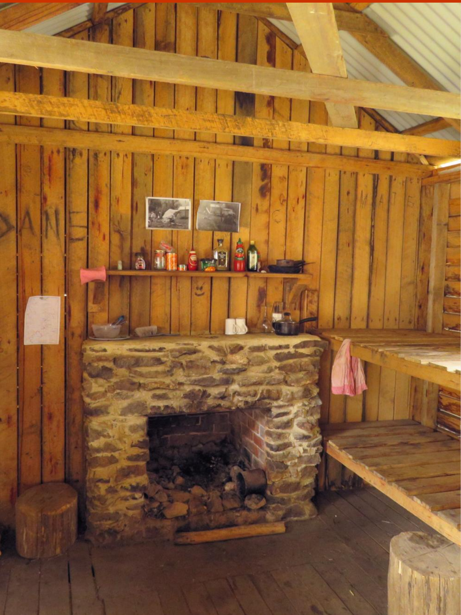
The inside of the hut is in excellent condition
