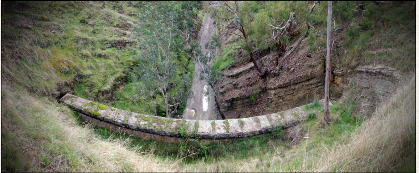
The west tunnel entrance from above 2012
