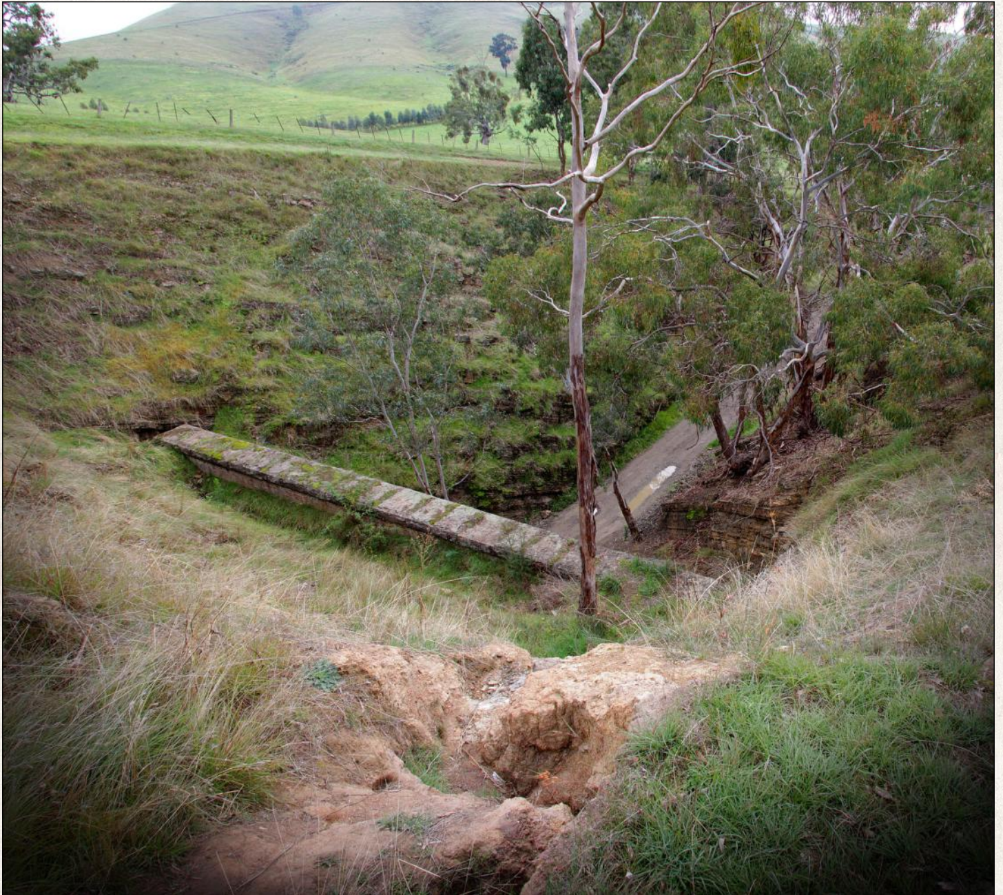
The west tunnel entrance from above 2012
