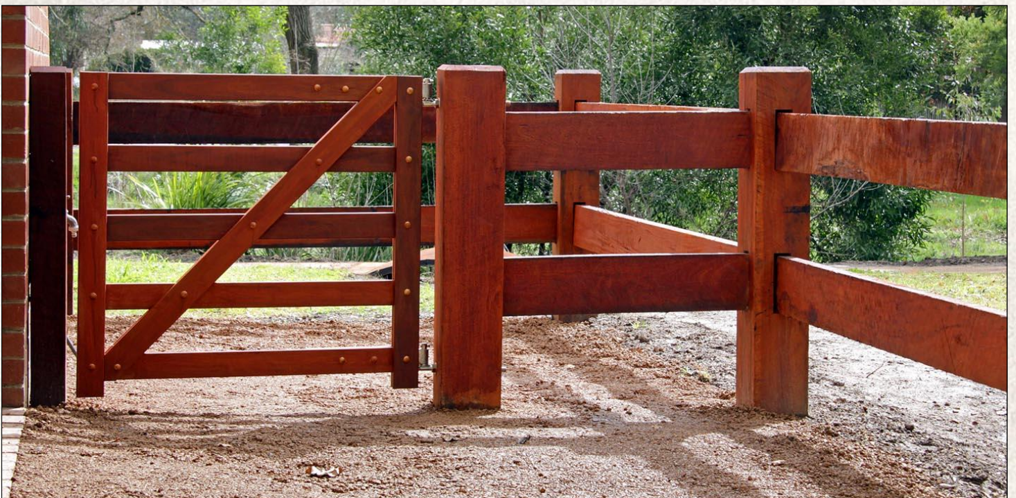
Taken during construction of the replica Red Gate August 2010.
