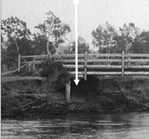
Bank collapse below southern approach to bridge
