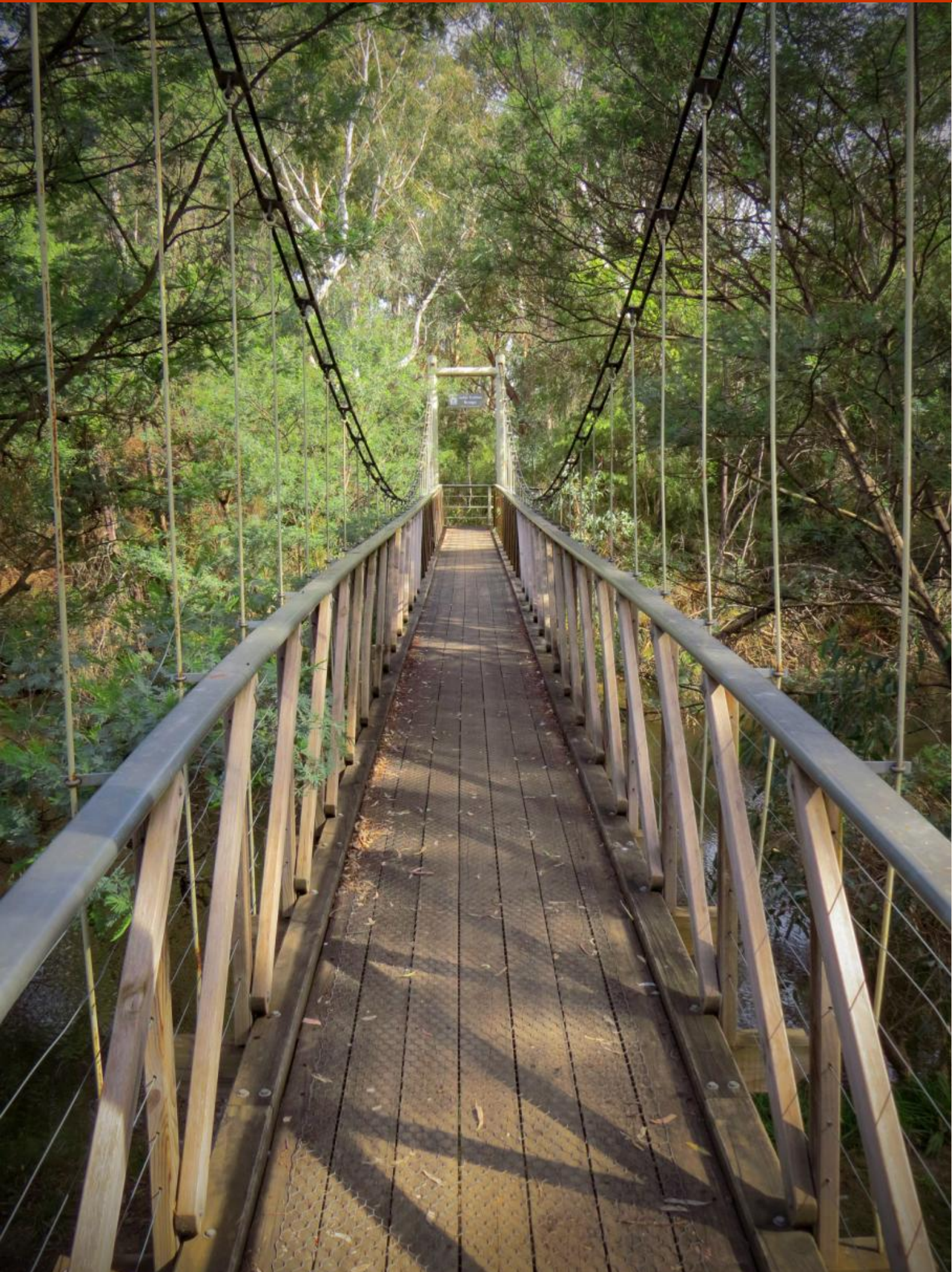
The Yea Wetlands Suspension Bridge
