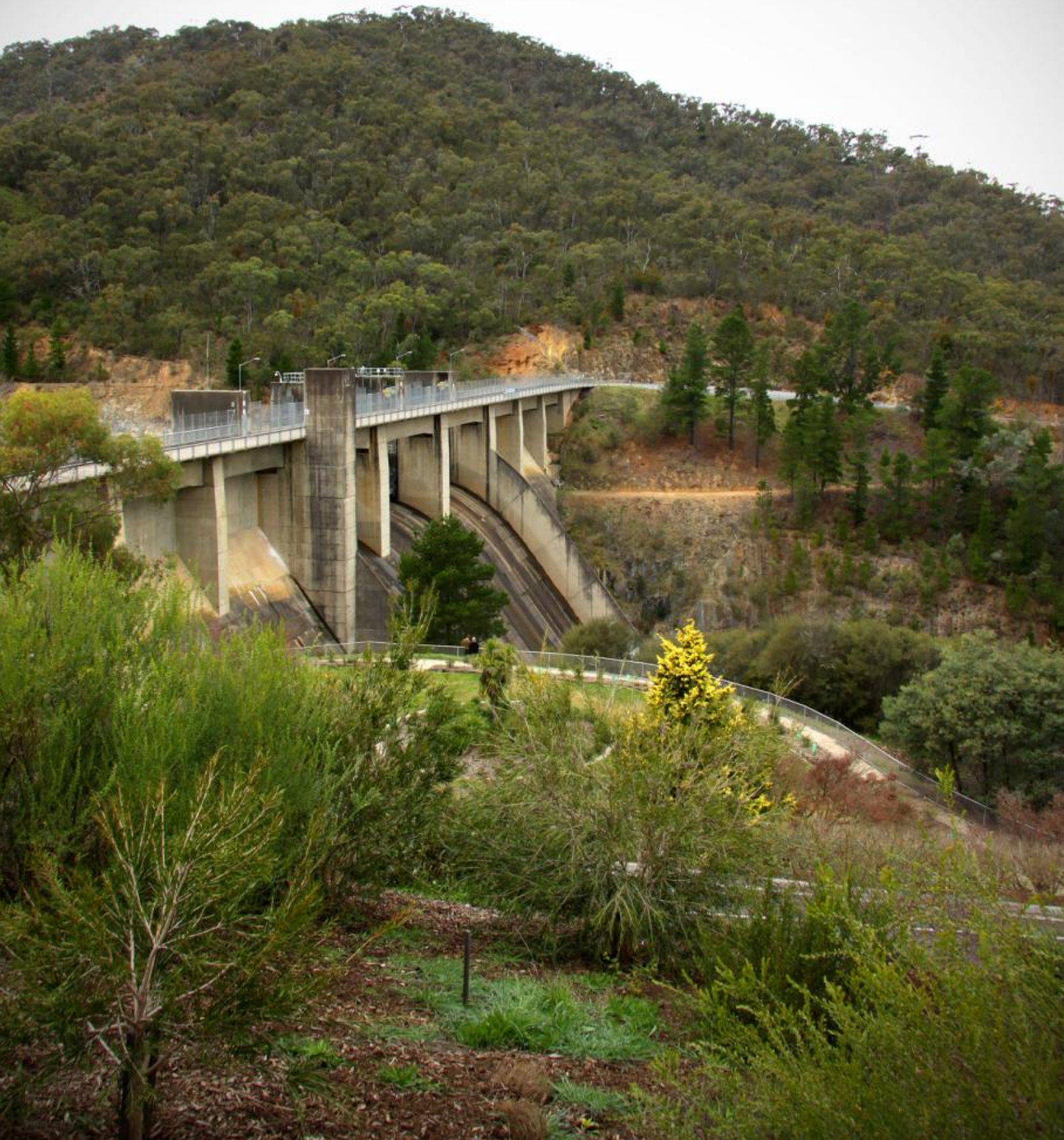
The spillway on Eildon Weir at Eildon.
