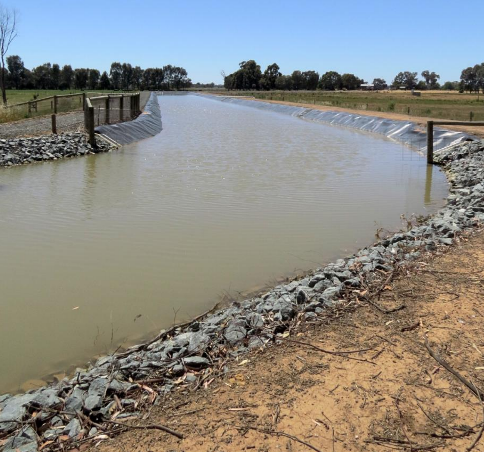
A government initiative to help reduce water loss by lining channels with plastic.
