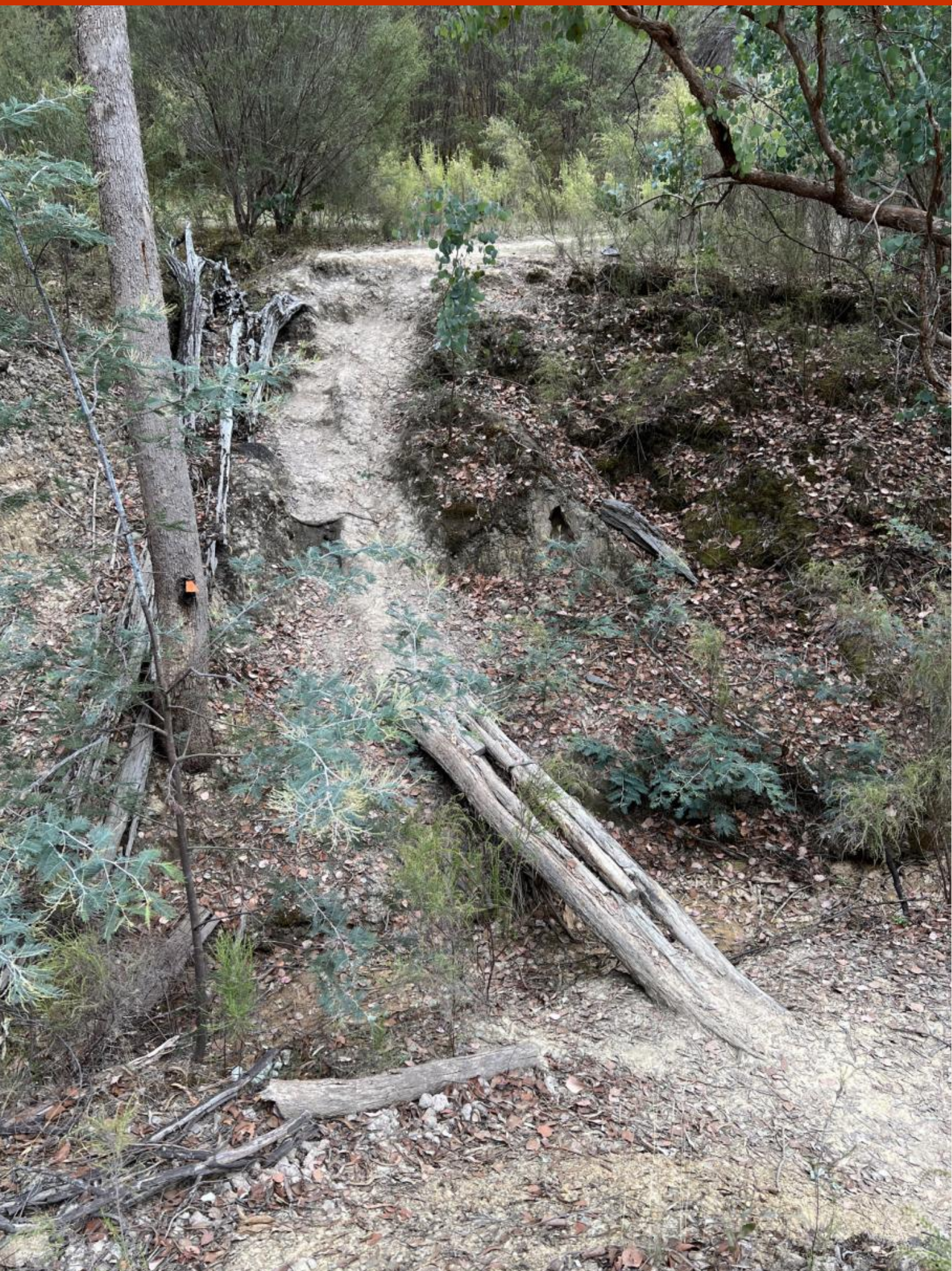
Tree trunks were used for this dangerous makeshift bridge
